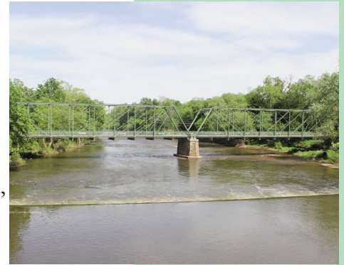
Nevius Street Bridge
