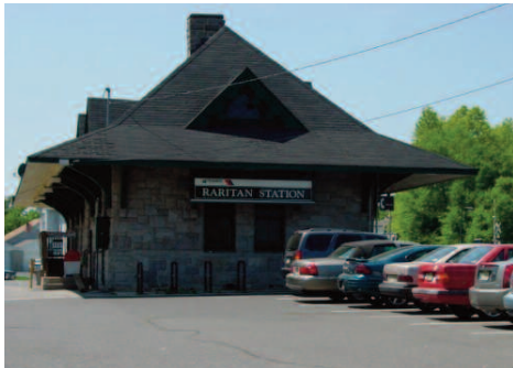
Raritan Train Station on the Raritan Valley Line
