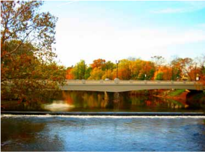
John Basilone Memorial Bridge
