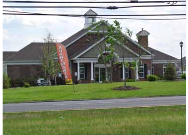
Stone Bridge at Raritan Residential Development
