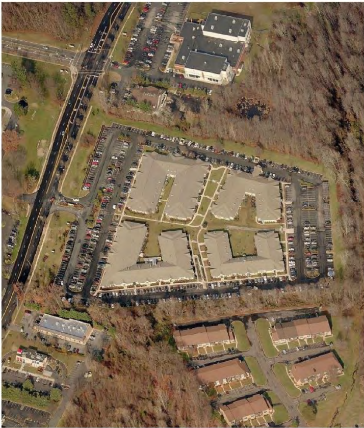
Top: Aerial of the existing Chimney Rock PGIA.
